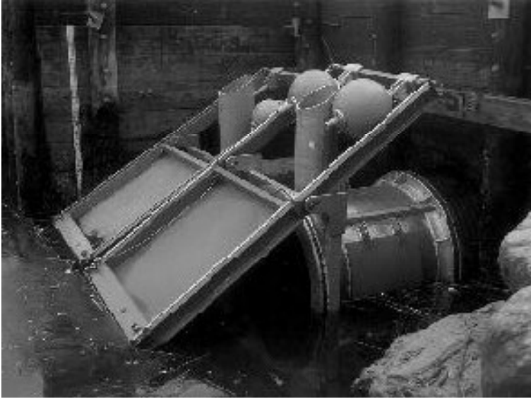
Photo 2- Self Regulating Tide Gate by Waterman Industries
