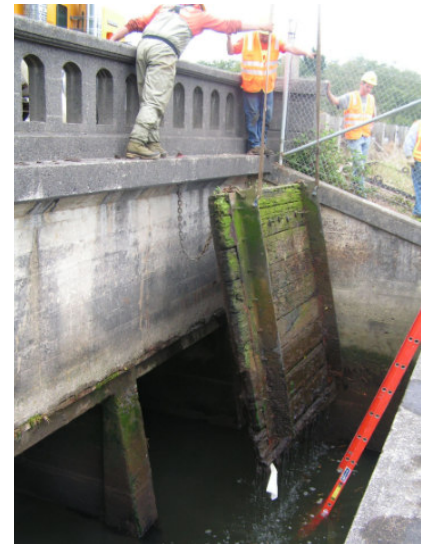
Photo 2 - Large timber flap gate
